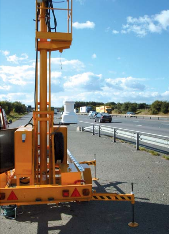
Left: Several different power and communications options open the way for Navtech Radar's systems to be used in portable ITS applications
